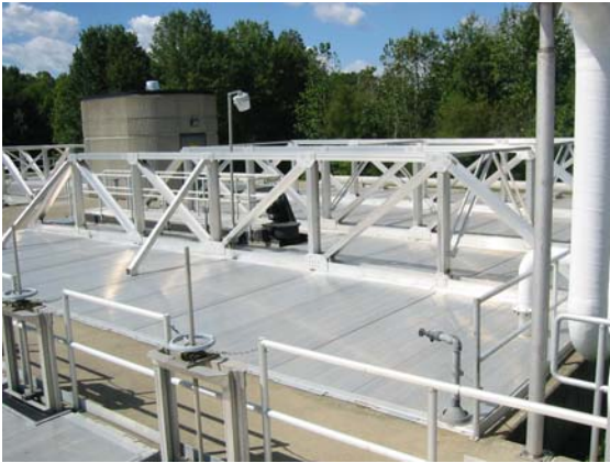
Examples of flat aluminum plate covers with external reinforcement
