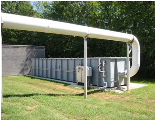
5,800 cfm biofilter by Biorem.
