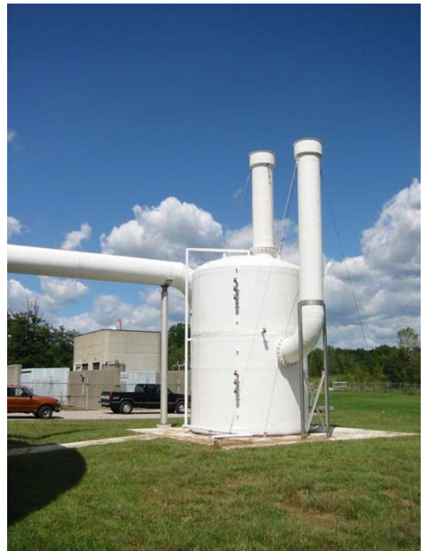
Existing 14,000 CFM Carbon Adsorber
