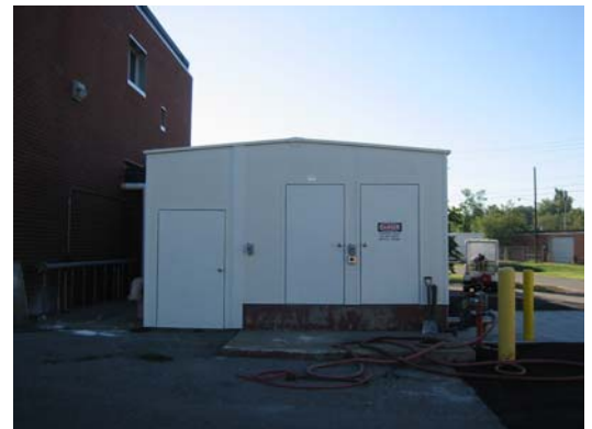
Enclosed Septage Receiving Station
