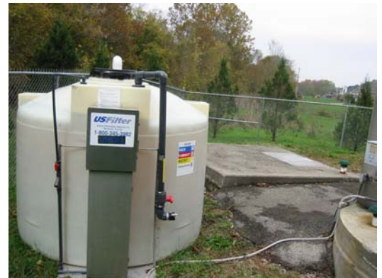
Typical Chemical Injection System
