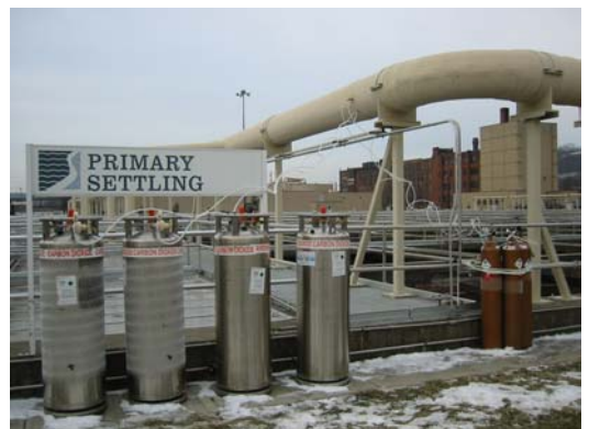
H 2 S & CO 2 Cylinders used in the testing
