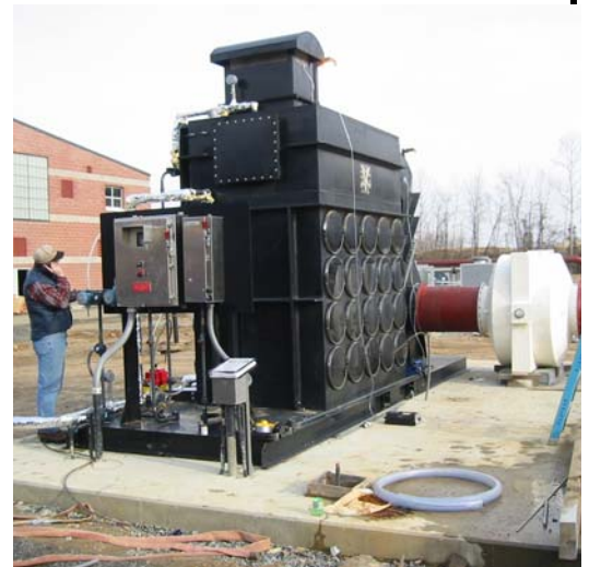
Carbon Adsorber (8,000 cfm)
