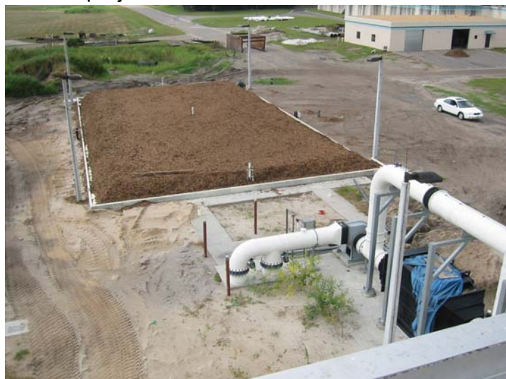
Existing Screening Structure Biofilter
