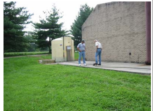
Route 108 PS and pilot chemical storage tank
