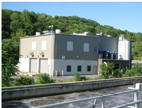
Downingtown WPCC Solids Handling Building
