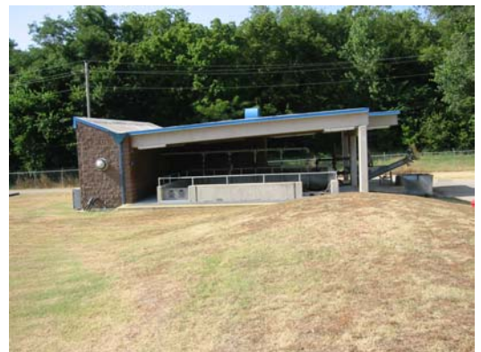
Aerated grit building
